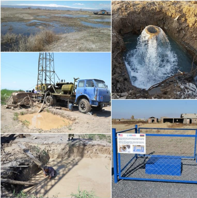
A photo collage of before and after photos and activities towards permanent sealing of the well.
