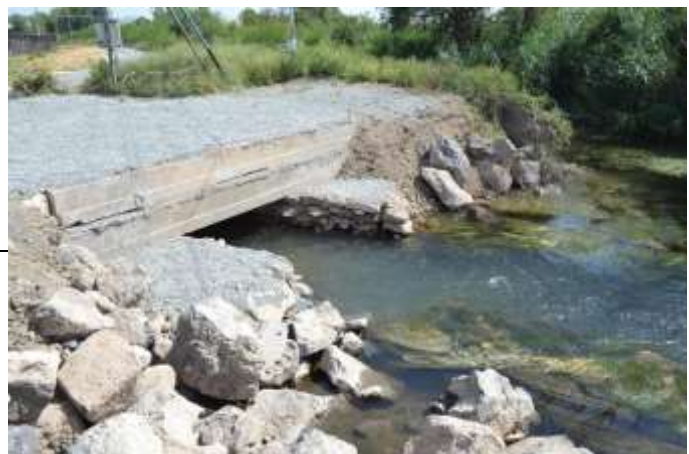
Reinforced drainage canal wall in the fish farm.
