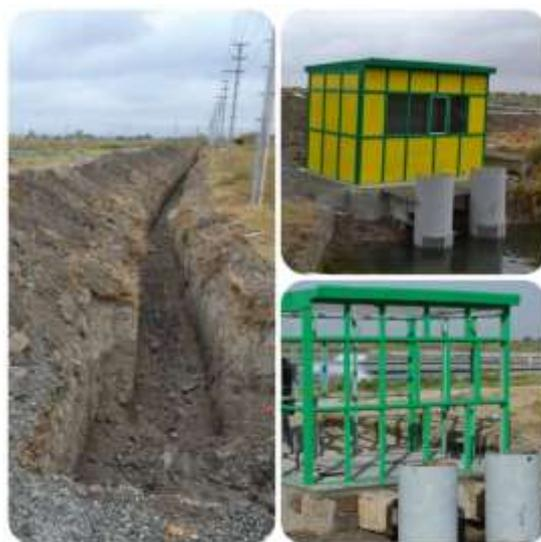
*The photo to the left: the trenches for the pipework to follow. To the right: the pumping station – semi-constructed and completed.*
