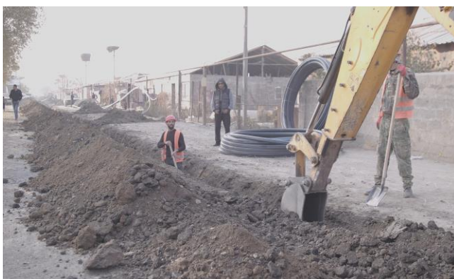
Installation of the irrigation network in Yeghegnut village.
