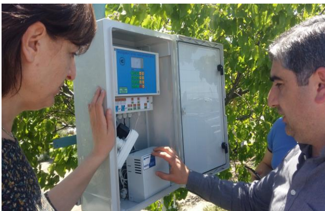
Flow-meters installed in Max Fish fishery.
