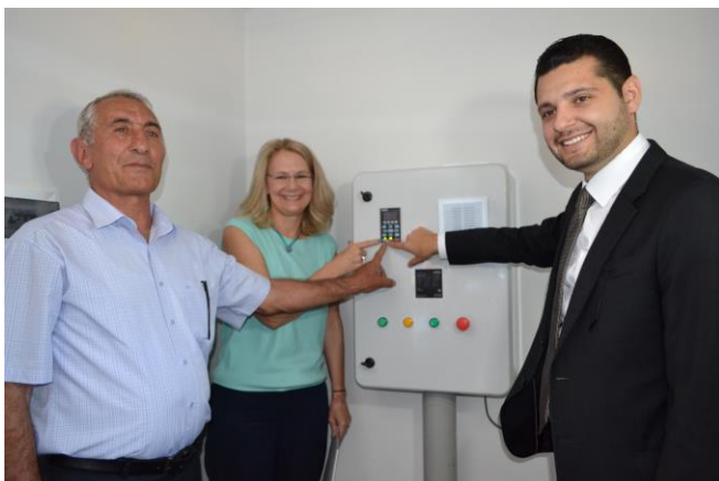
USAID Mission Director Deborah Griser, mayor of Aratashen Vahram Harutyunyan (on the left), and Governor of Armavir region Hambarzum Matevosyan (on the right) launch the newly installed pump in Aratashen.
