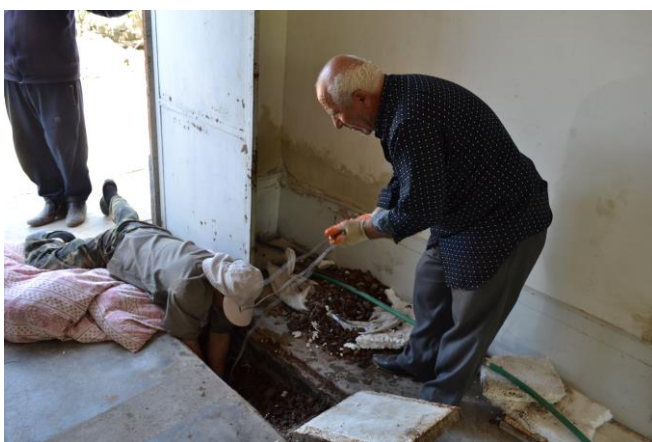
Installation of household network in Aratashen
