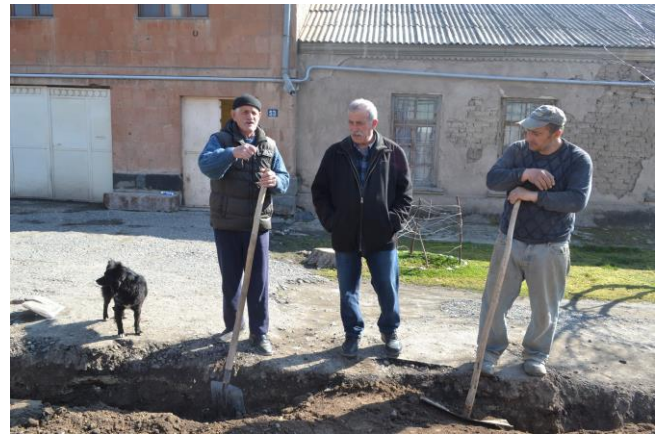
Village residents backfilling the trenches near their homes.
