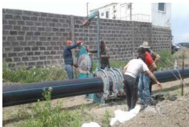
*Left to right: construction of the ATTC premises and installation of irrigation pipes in Sayat-Nova village.*
